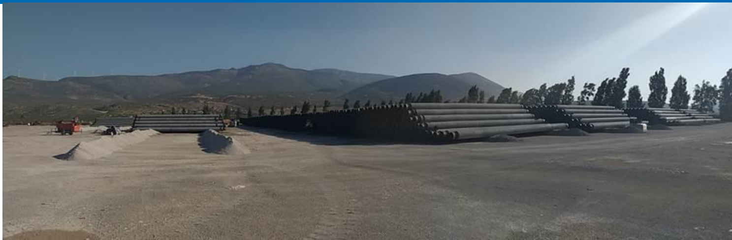
○ MCS Build (99% completed)
