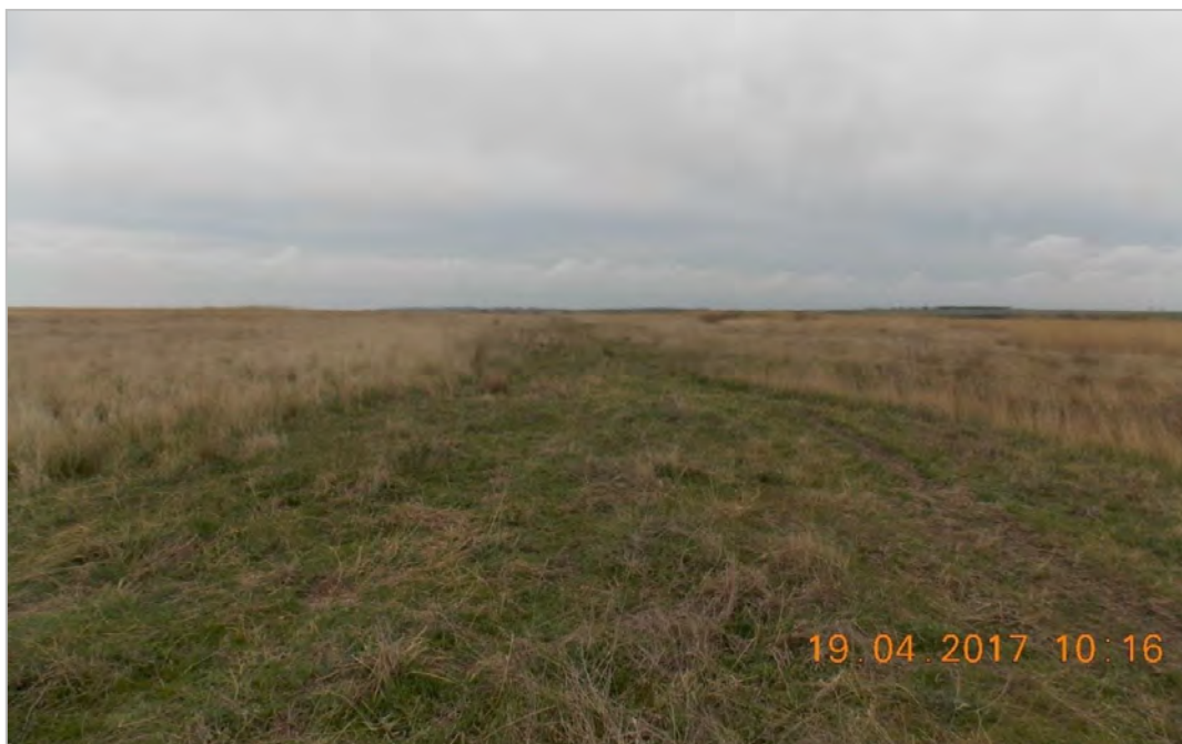
Photo 5.1 Route portion of the underground onshore pipeline (view from west towards east)
