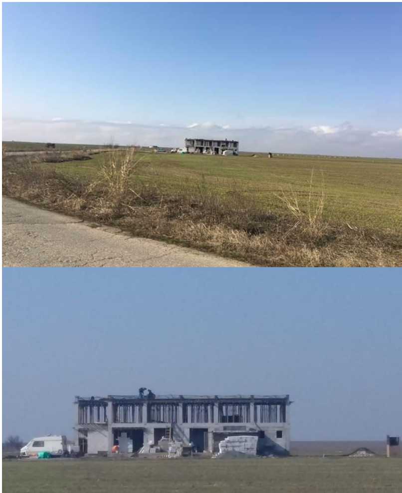
Figure 9-7 - Guest House under construction in Vadu (February 2019)
