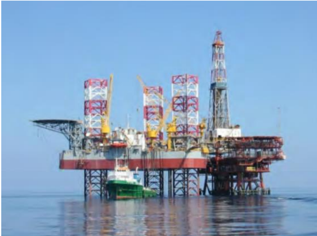
Figure 0-6 GSP Uranus jack-up drilling rig
