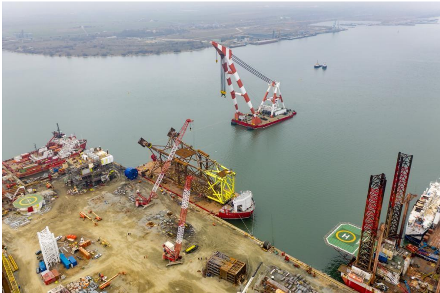
Picture 1 Ana platform - Jacket load out - Agigea
