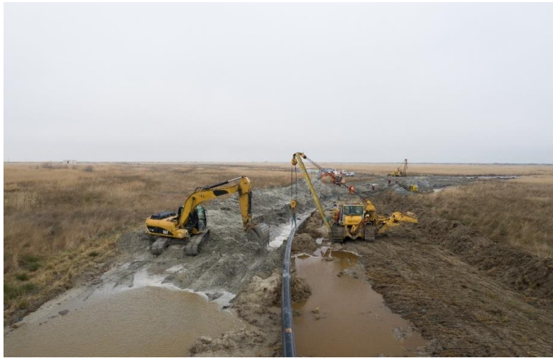
Picture 6 and 7 Pipeline laying in Vadu
