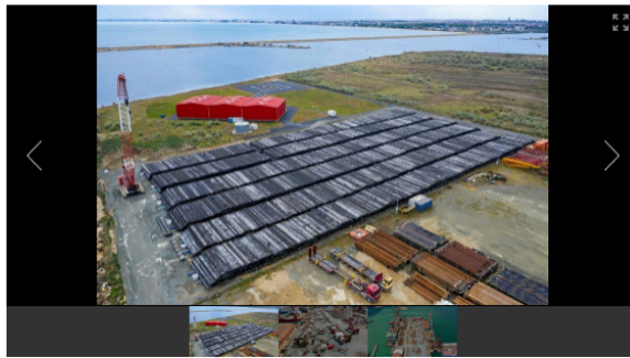
Work progress: pipe storage in Midia base Photo: BSOG
